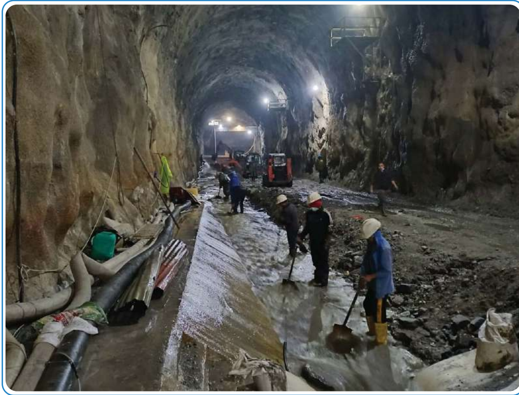
Desander Basin Debris Clearing
